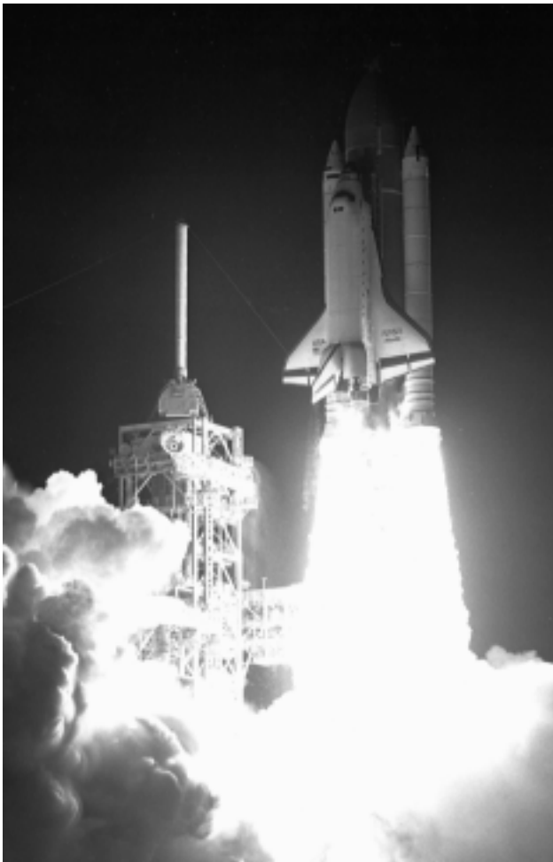
The light from the liftoff of the Space Shuttle orbiter Atlantis on mission STS 61-B highlights Launch Pad 39A's lightning mast and attached Catenary Wire. The mast and wire provide the primary lightning protection system for the orbiter while it is on the pad.
